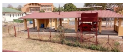
Figure 7. The operational incinerator installed by MSF and the newly installed by WHO.
